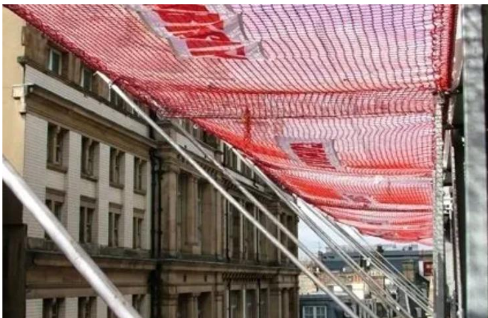
Figura 4.3-1 - Safety net fan (Combisafe)
