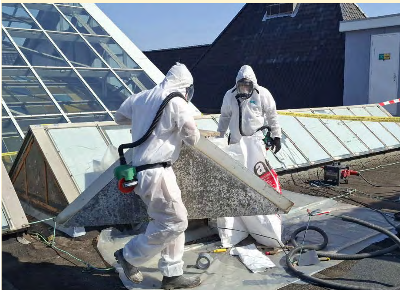
Figure 4-4: Workers removing asbestos plates on the roof
