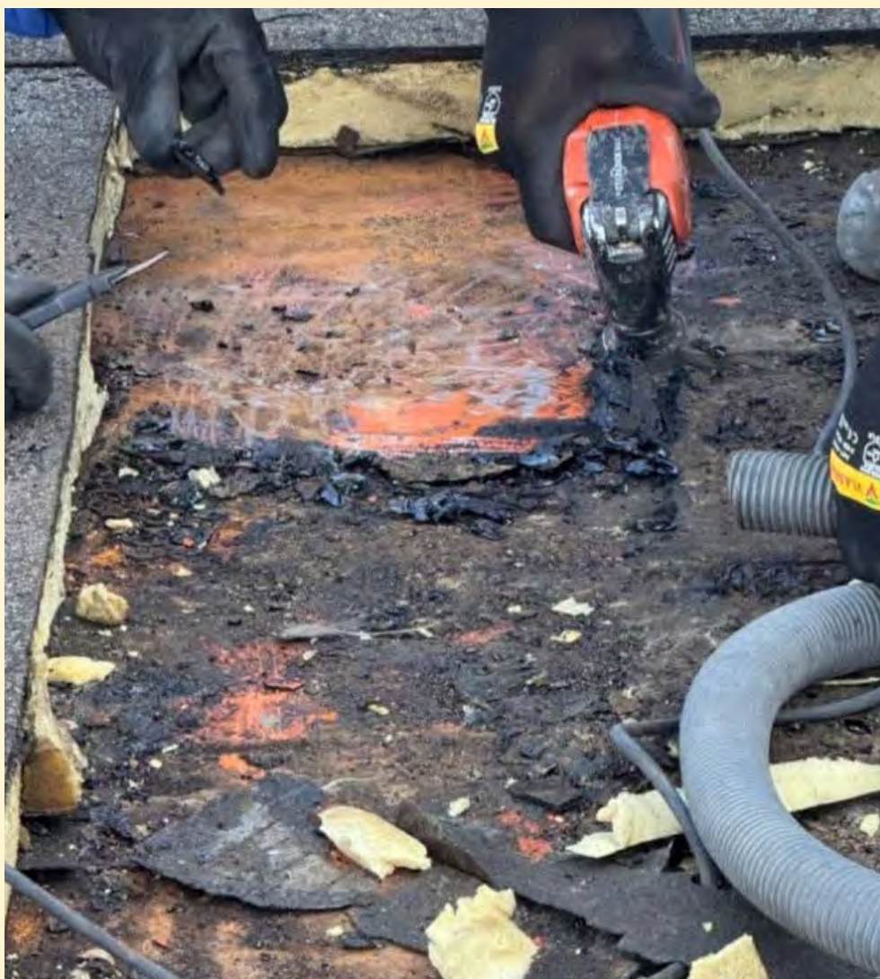
Figure 4-3: Removal of roofing materials containing asbestos, with metal supportive roof visible
