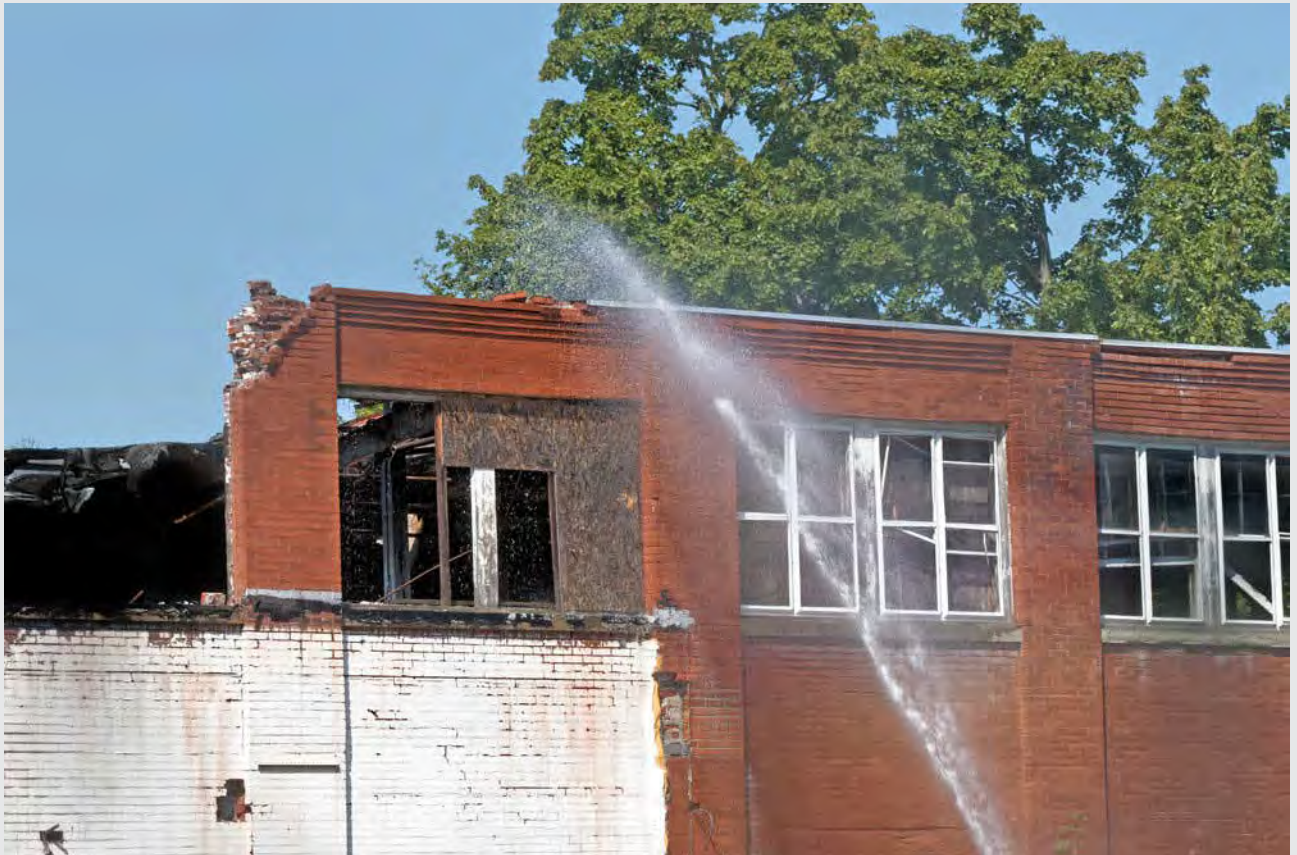
Figure 8-1: Example of wetting a building containing asbestos
