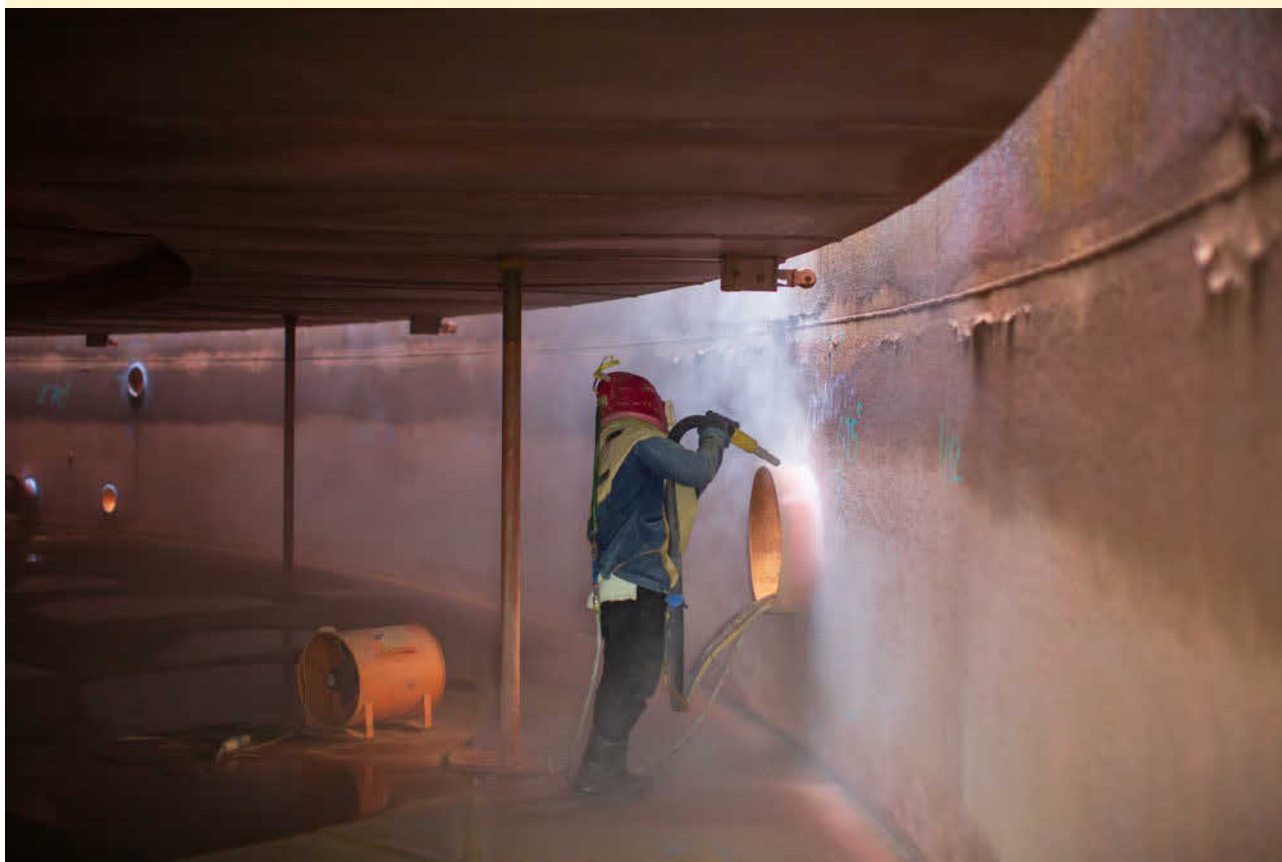
Figure 11-1: Worker removing paint inside of a fuel storage tank using blasting grit
